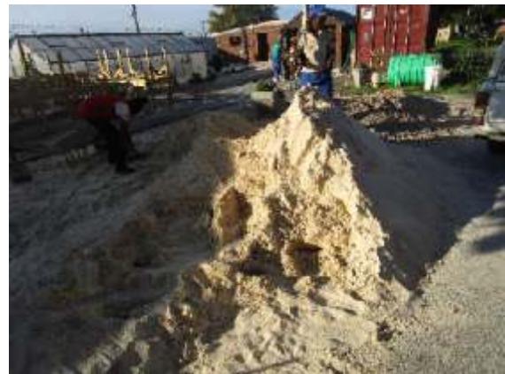
Sand preparation for pavers.
