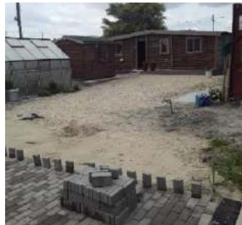
Paving and edging underway.
